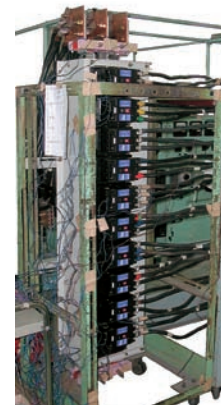
Status of multi-step temperature test
