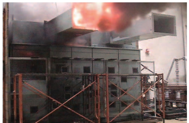
Arcing due to internal fault test
