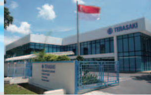
TERASAKI CIRCUIT BREAKERS (S) PTE. LTD. TERASAKI ELECTRIC CO., (FAR EAST) PTE. LTD. (シンガポール)
