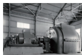
The first generator for short-circuit tests
